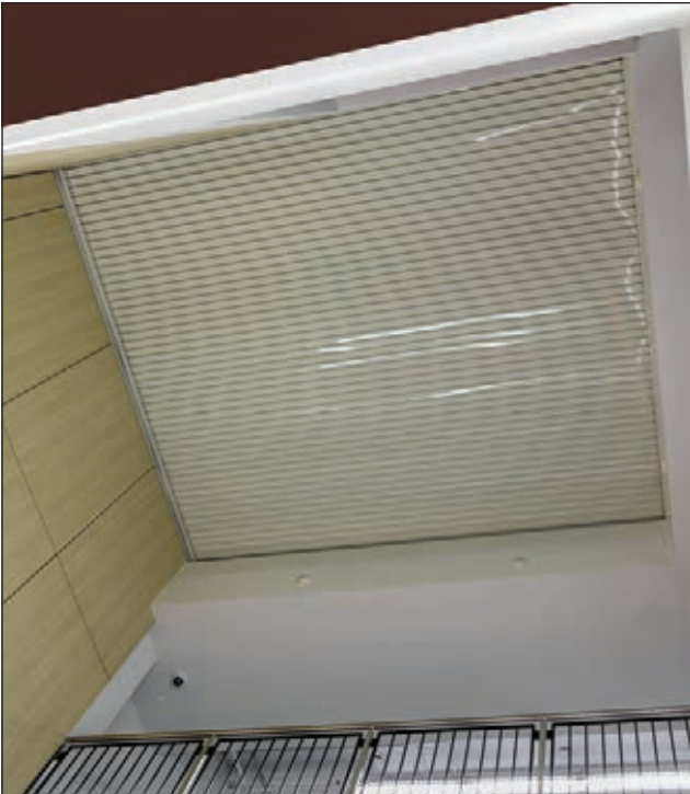
UL 10B 2-hour & UL 1784 “S” labeled, hose stream tested assembly.
