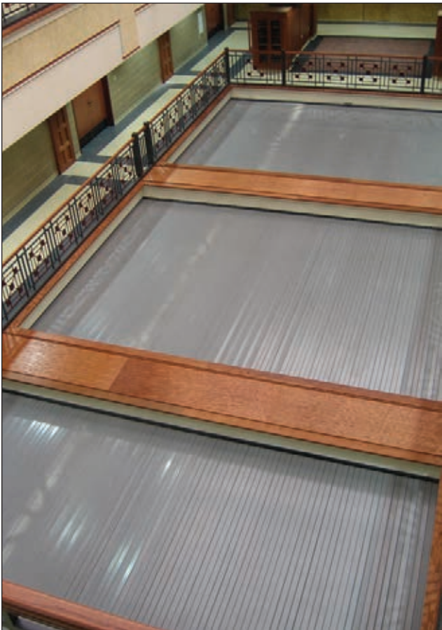
UL 10B 2-hour & UL 1784 "S" labeled, hose stream tested assembly.
