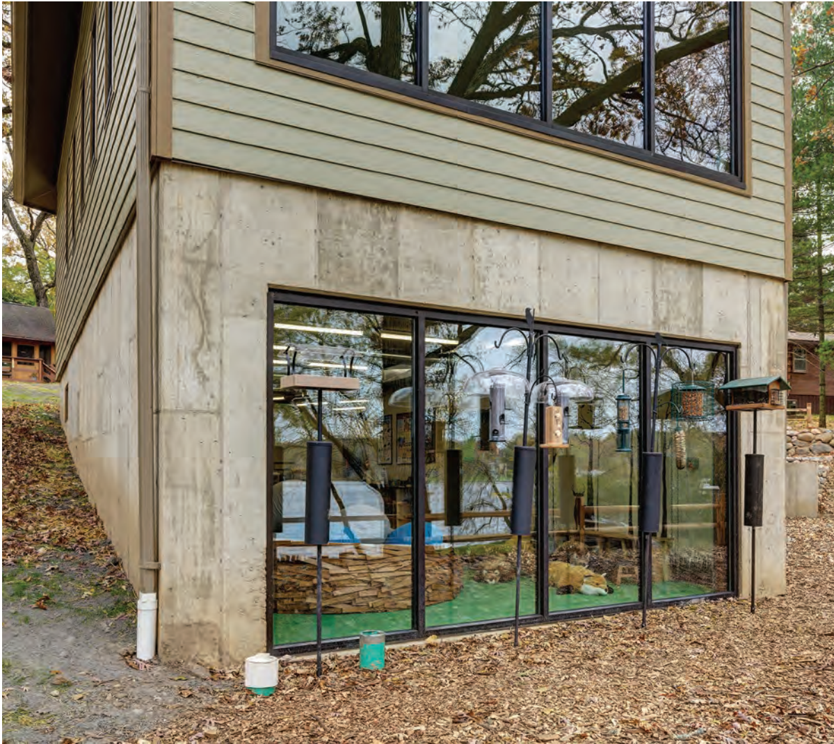
SafeSpace™ 500 | Valerie Hall Outdoor Education Center
