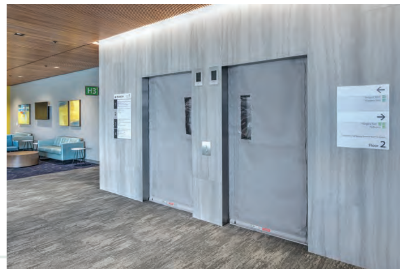
SmokeFighter Model D150E is available with an ASME A17.1 compliant vision panel when required.
